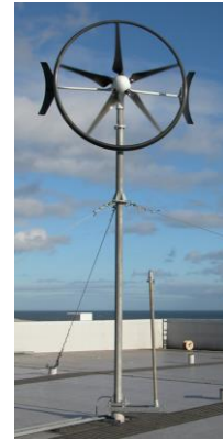
Figure 4 - Swift 1.5kW wind turbine
