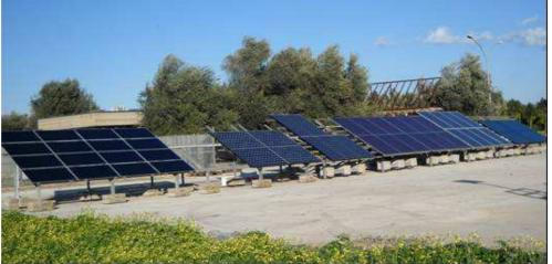
innovative PV systems (usually from 1 to 20 kW peak power), using accurate data acquisition tools (developed by RSE) for analysis of DC and AC electrical parameters, in-site environmental data and evaluation of performance yields and reliability.
