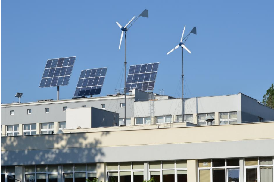
Photograph: Sun tracking system and wind generators (DER laboratory at TU Lodz)
